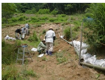
畑の法面補修
